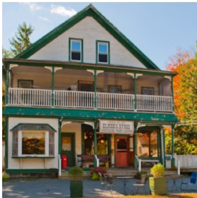
Sidewalk café in Ashfield village center
