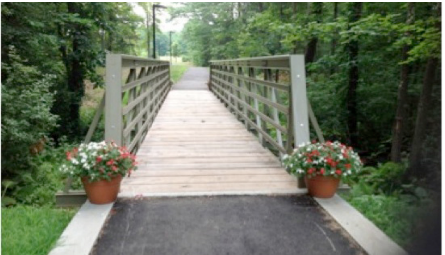
Boxborough's innovative fiberglass pedestrian bridge
