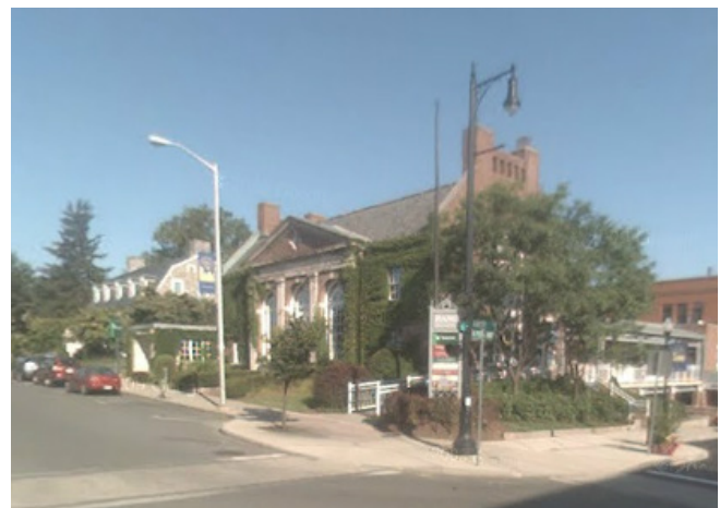
Curb extension in Amherst
